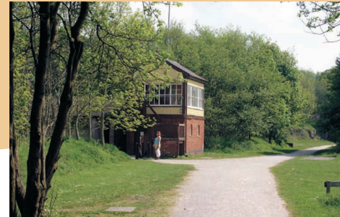
Hartington Signal box
